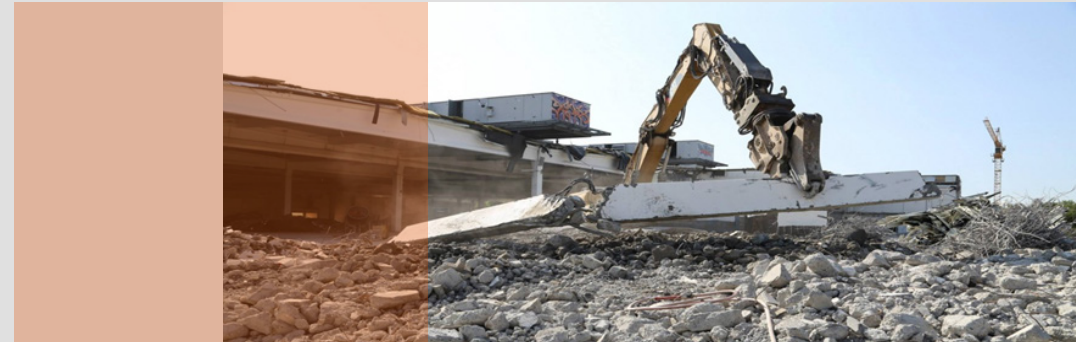
fig.9: dismantling Exchange shopping mall
