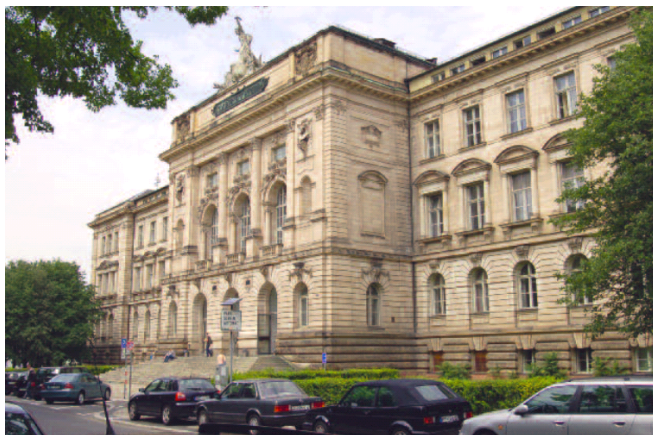
The university building at Sanderring in the city center.
